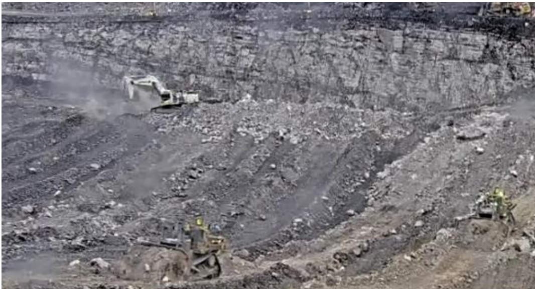
Figure 6. A small digger side cutting highwall
