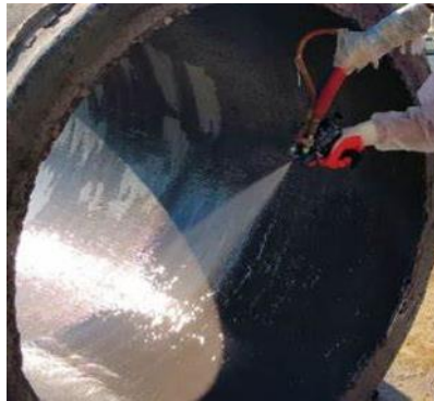
Photo 6. Epoxy spraying
