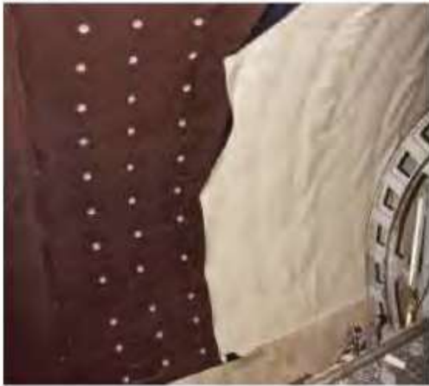
Figure 7. DELTA®-AT 1200 and the yellow waterproofing membrane
