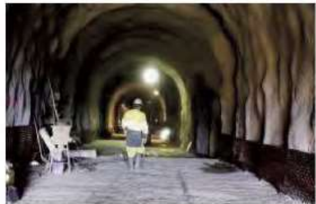
Figure 17. Inside of the tunnel
