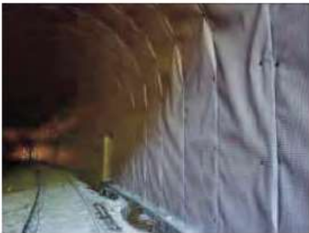
Figure 25. DELTA®-PT installed
