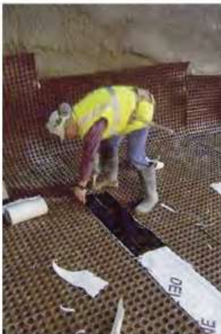
Figure 19. DELTA ® -THENE strips
