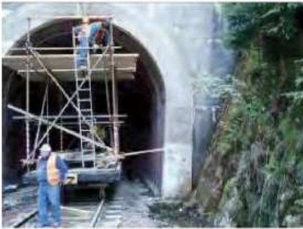
Figure 24. Nové Hamry railway tunnel
