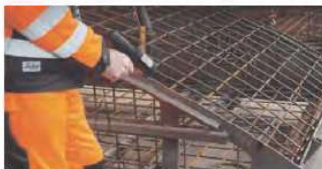
Figure 6 Segment reinforcement scan
