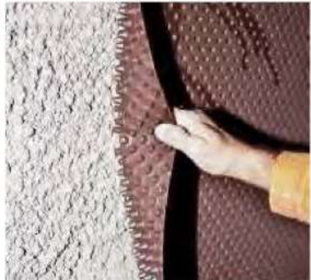
Figure 9. DELTA®-AT 1200 and shotcrete
