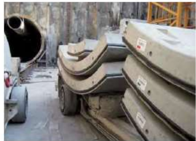
Figure 4. Segment bar-code identification
