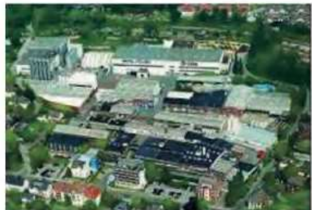
Figure 1. Dörken Factory in Herdecke, Germany
