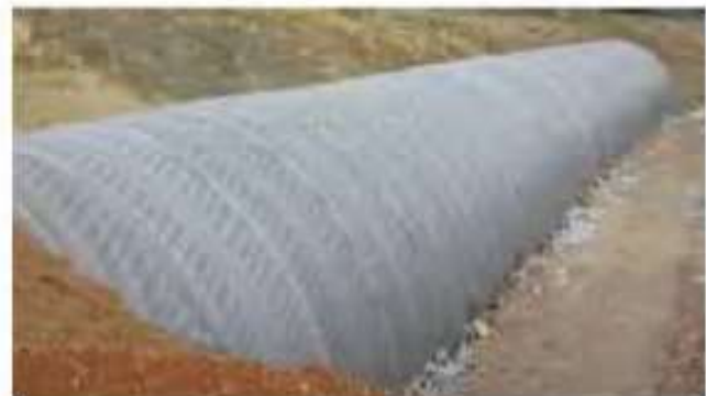
Figure 28. DELTA®-TERRAXX application in Kemalpaşa Tunnel project
