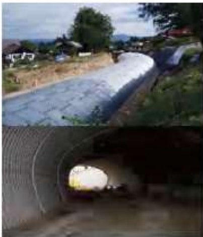
Figure 2. Plan view of the corrugated steel structure and inside view prior to shotcrete
