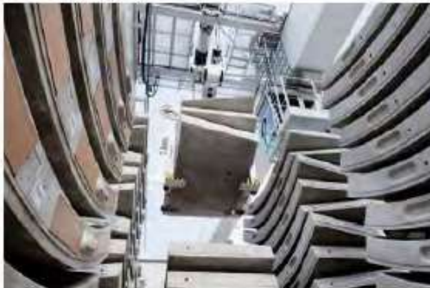
Figure 7. Koralm storage area
