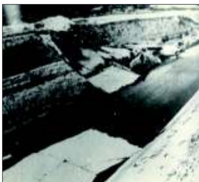
Figure 1. Example of disorders in the construction of « Samour –Apcheron » concrete channel.
