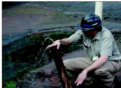
Figure 3: Drainage control by piezometers
