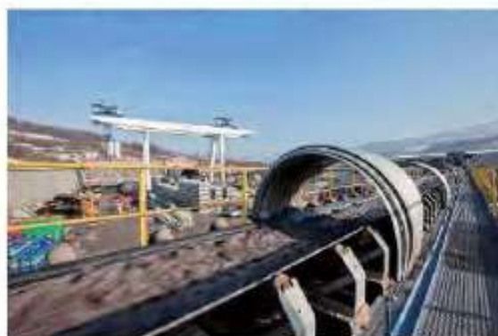
Figure 4. Excavated soil conditioned on conveyor belt
