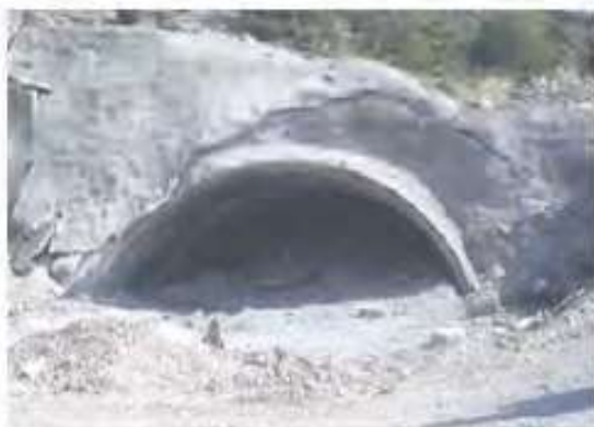
Figure 1. Abandoned NATM Tunnel prior to alignment change
