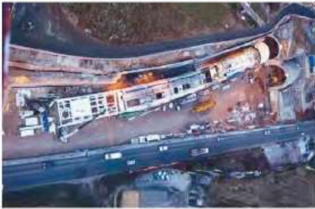
Figure 6. General view of the TBM
