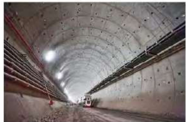
Figure 8. Sparvo tunnel completed
