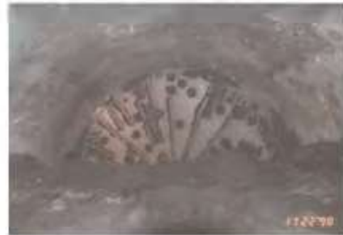
Figure 1. Entrapped TBM in Pinglin tunnel
