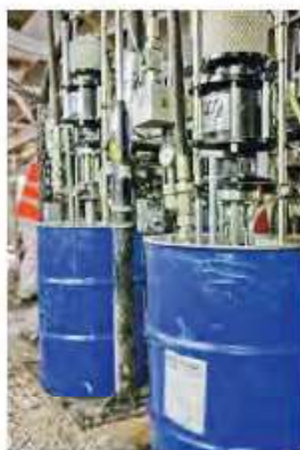
Figure 5. Suction of tail sealant MasterRoc TSG 6
