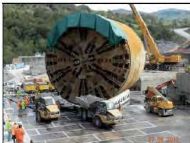
Figure 5. U-Turn of the shield
