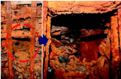
Fig. 12 Cavity by rock fall
