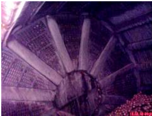
Figure 6. Inside view of Esfordi ball mill showing discharge grate
