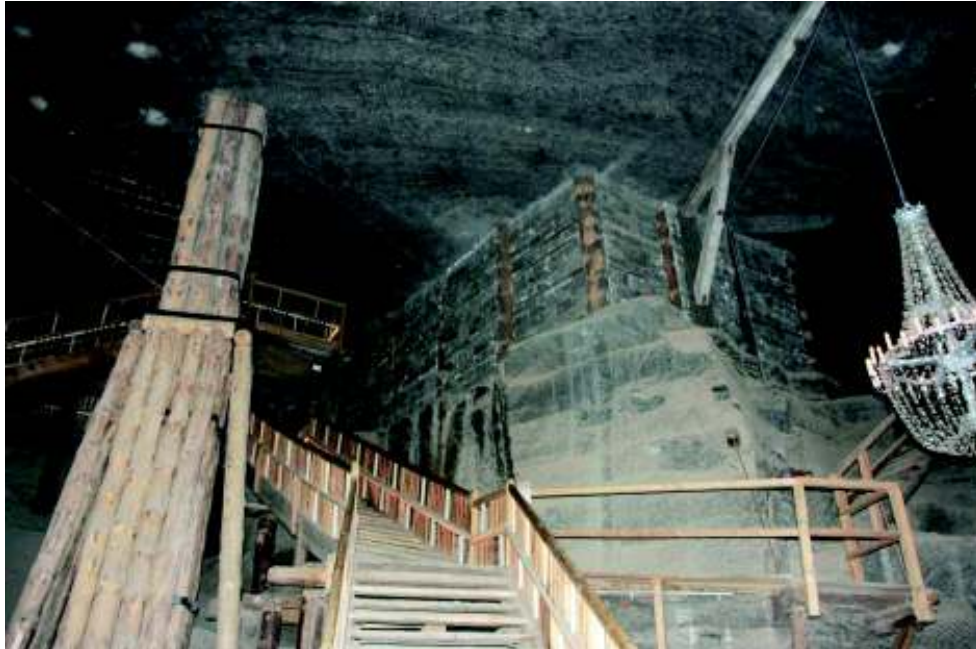
Figure 16 Supported salt roof strata in Saurau cavern
