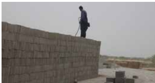
Fig. 8. A man watering the concrete blocks made at the mining site.
