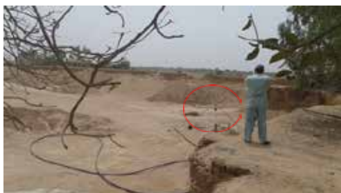
Fig. 7. Showing drilling of percussion well in bed rock (Gaj Formation)
