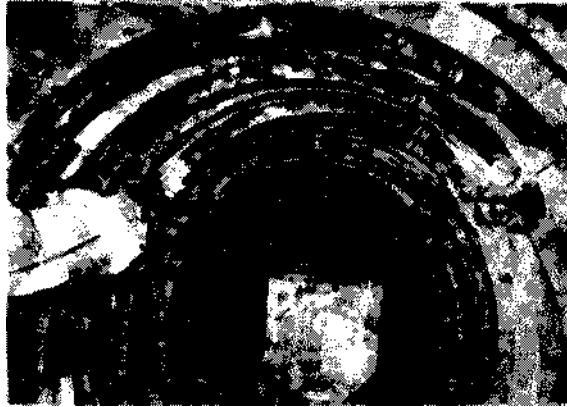
Figure 4. Bateway elliptic yielding supports
