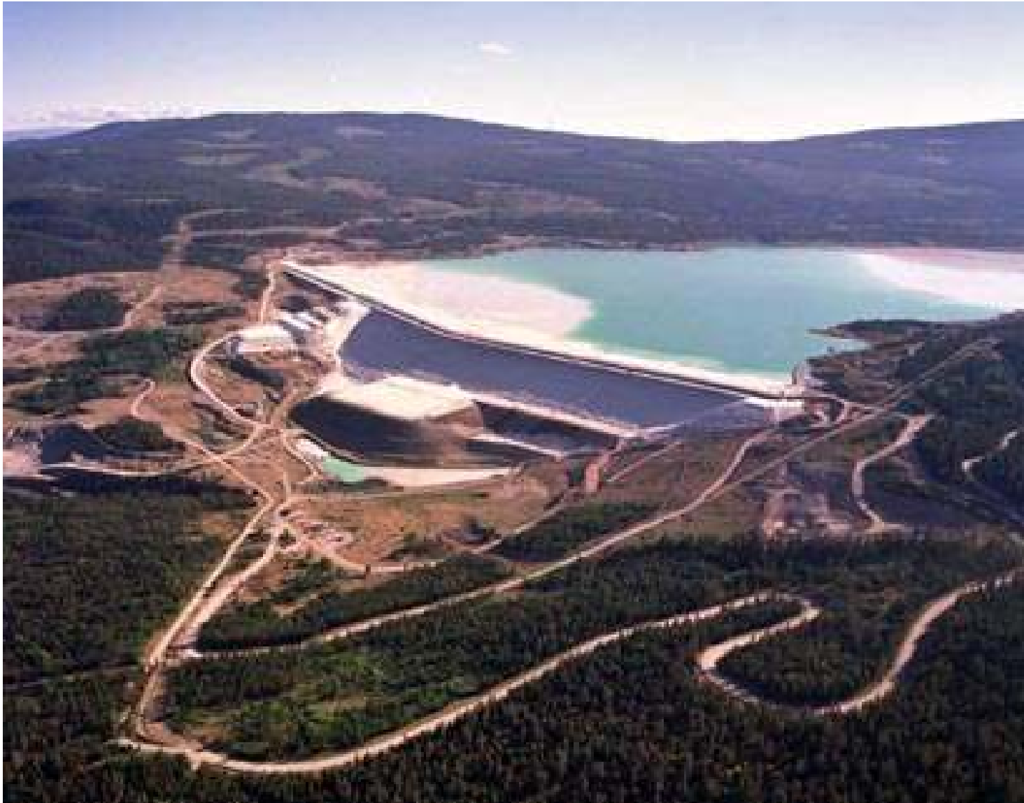
Figure 4: Cross valley tailings impoundment at Highland Valley Copper, BC, Canada (Courtesy TeckCominco)
