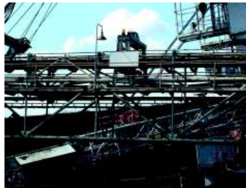
Figure 7. On-belt Ash-analyzer on the discharge boom of a bucket wheel excavator
