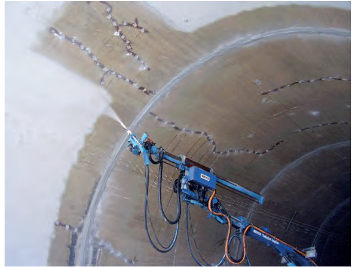
Figure 2. TSL application for the aim of water resisting (Wallis, 2008)
