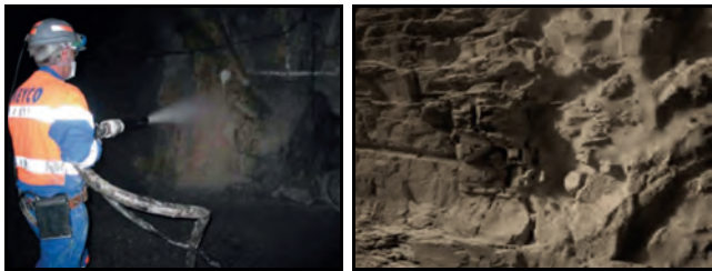
Figure 1. Application of TSL Product (BASF, 2013).
