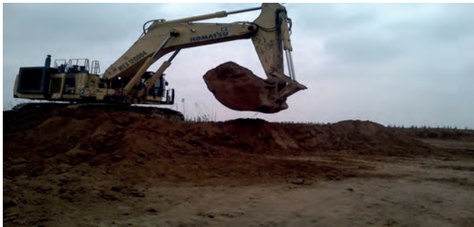
Figure 5. Excavator in the pit waiting for truck
