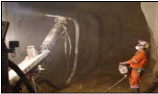
Figure 1. Application of Shotcrete
