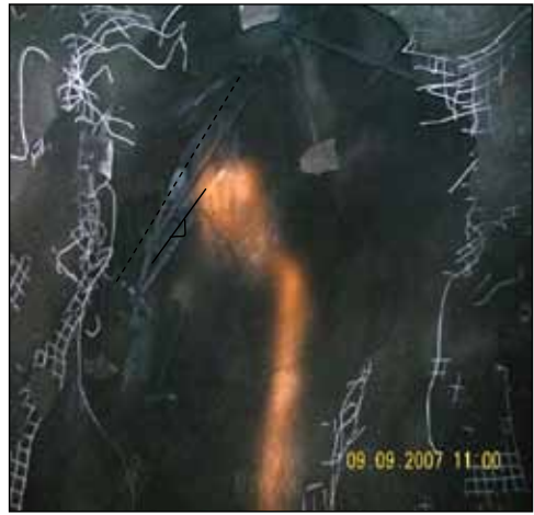
Figure 3. Rockfall cause form sliding plane (Geotech: 2007)
