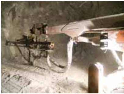
Figure 5. detail of a Tamrock jumbo while performing the drill-holes.
