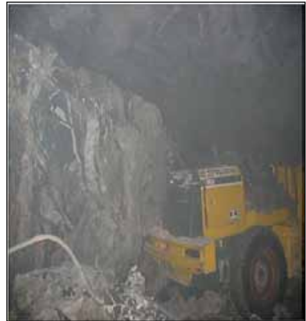
Figure 1 Rockfall cause form slabbing with equipment damage (Geotech: 2007)
