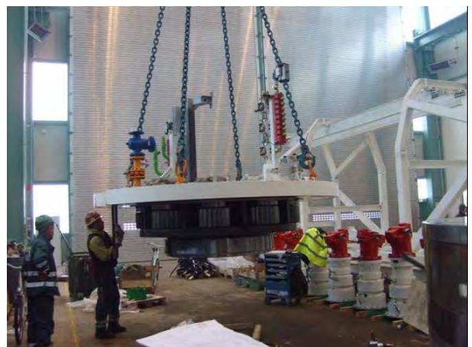
Figure 1. The main drive of the TBM
