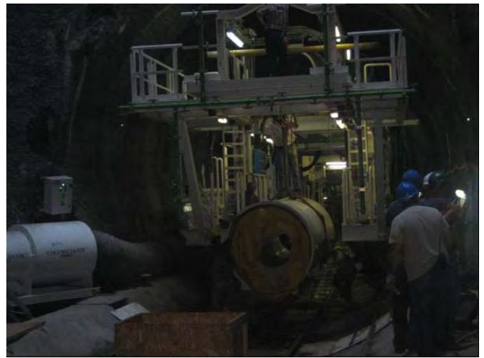
Figure 12. Assembly of the air duct on gantry 5
