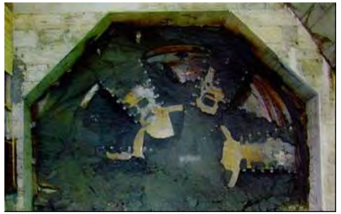
Figure 9. Clean cutterhead after breakthrough
