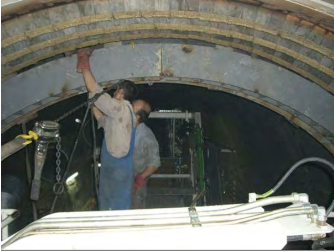
Figure 14. Adjustment of the thrust ring
