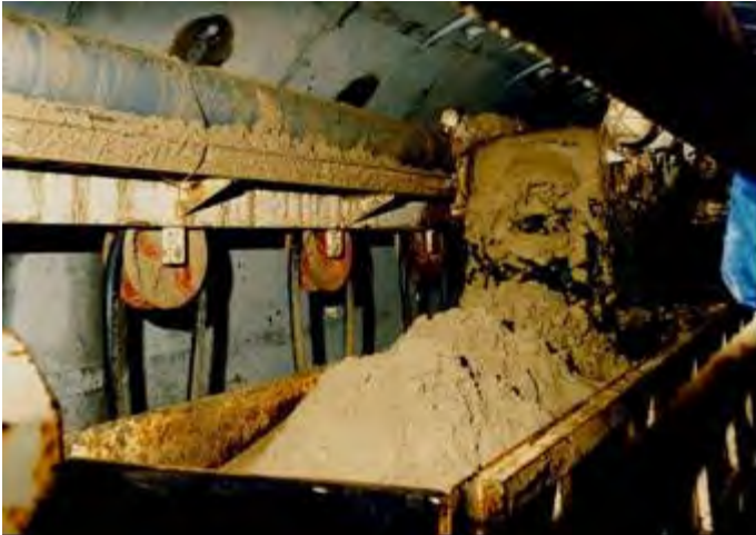
Figure 8. Sand excavation with Foam and Polymer
