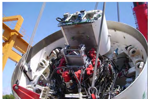
Figure 3: Shield lifted with an angle
