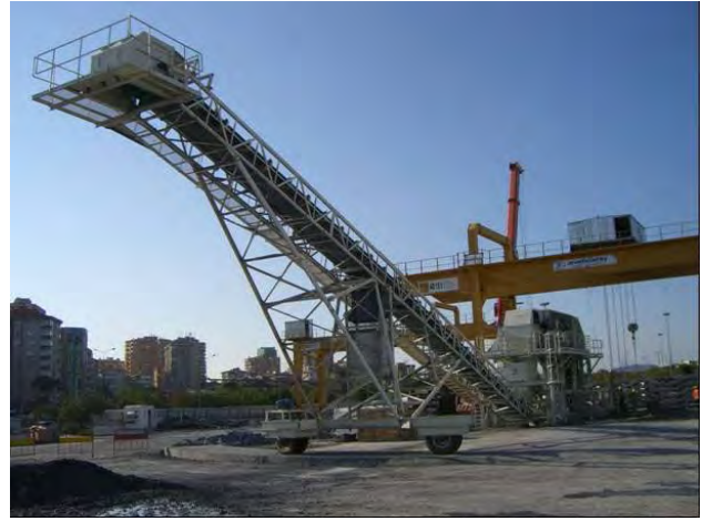
Figure 18. The place where the muck is loaded inside the trucks
