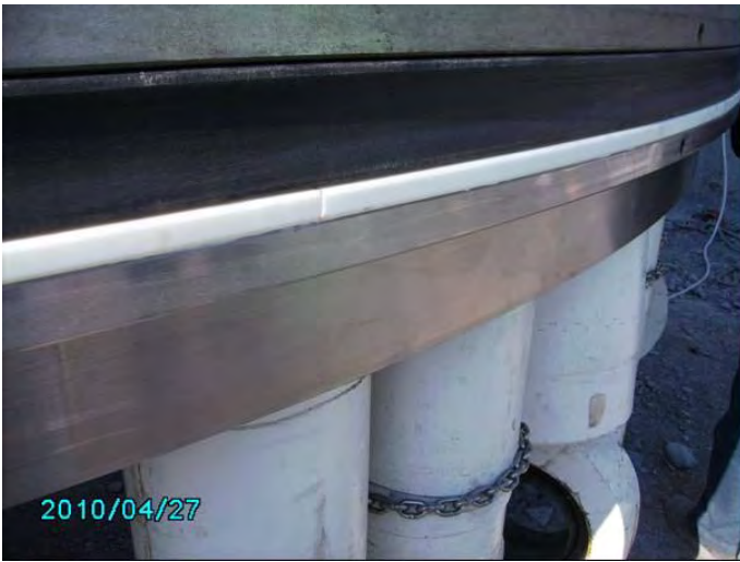
Figure 4. Sealing set with the support system
