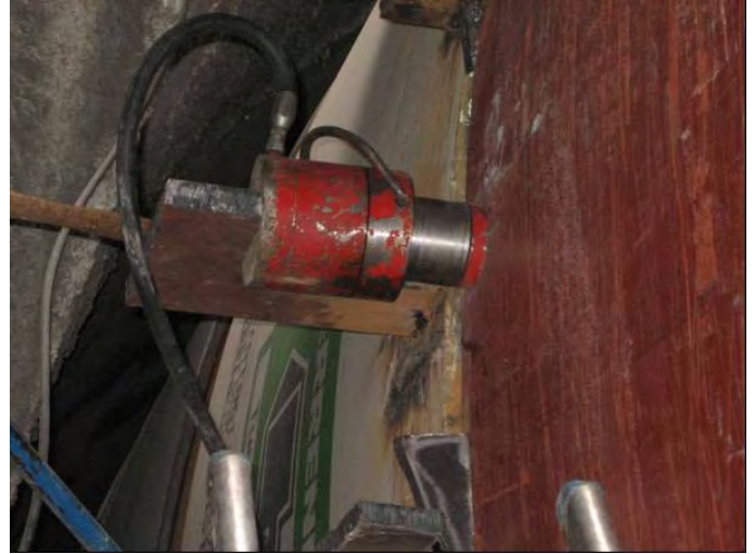
Figure 7. Adjustment of tailskin with the hydraulic cylinders and steel plates
