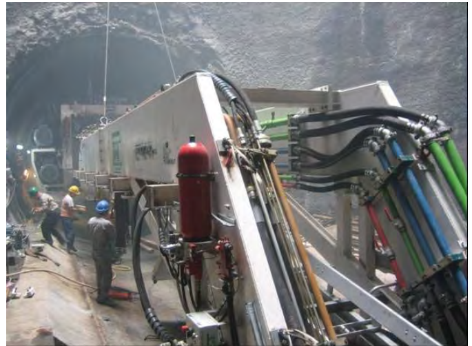
Figure 10. Bridge lowered down inside the shaft
