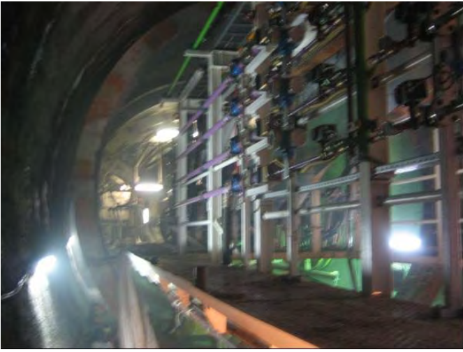
Figure 11. Thrust ring welded on the bridge
