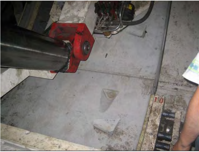
Figure 16. An example of ring building
