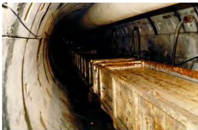
Figure 7. Sand excavation only with foam
