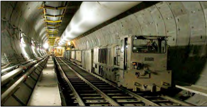
Figure 4. TBM support logistics have a very important impact on TBM performance.
