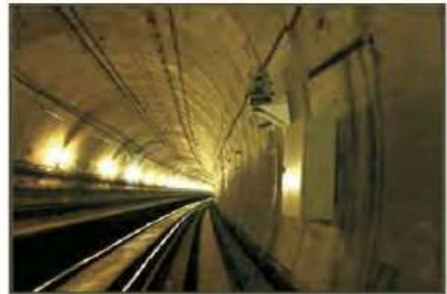
Figure 9. Automated geodetic system Cyclops performing 3D real-time measurements in running tunnel
