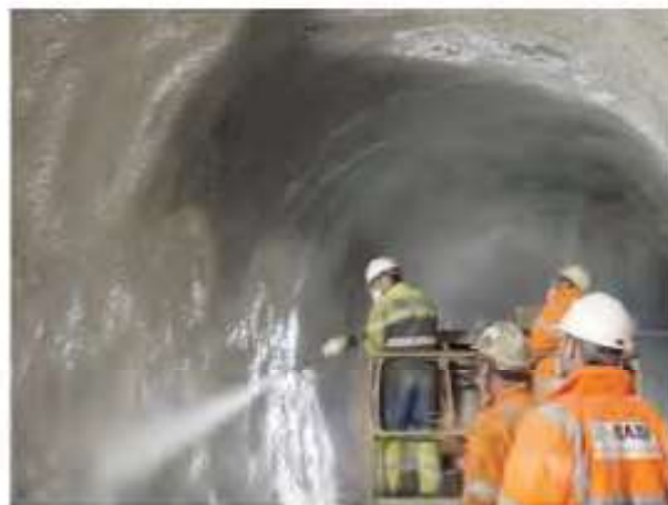
Figure 11. Membrane application in the cross passage of the Hindhead Tunnel, UK
