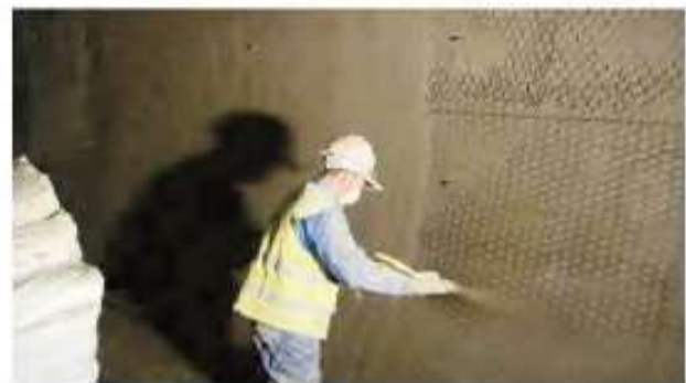
Figure 17. Second coat spraying
