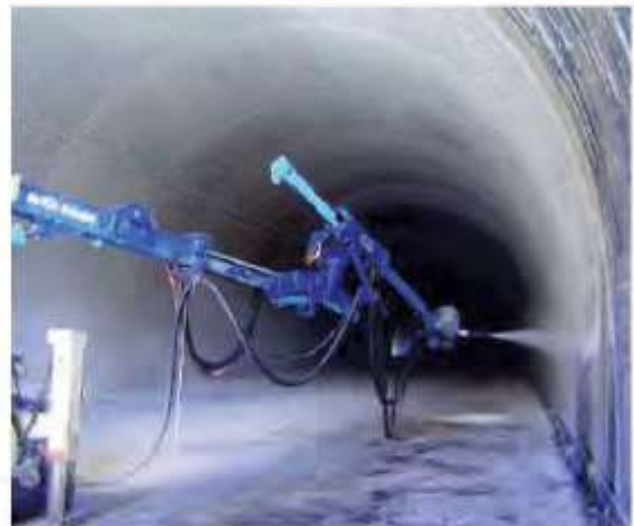
Figure 13. Robotic membrane application
