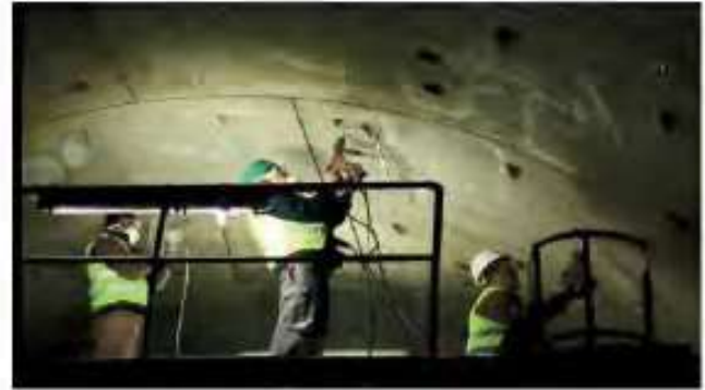
Figure 13. Drilling for anchors
