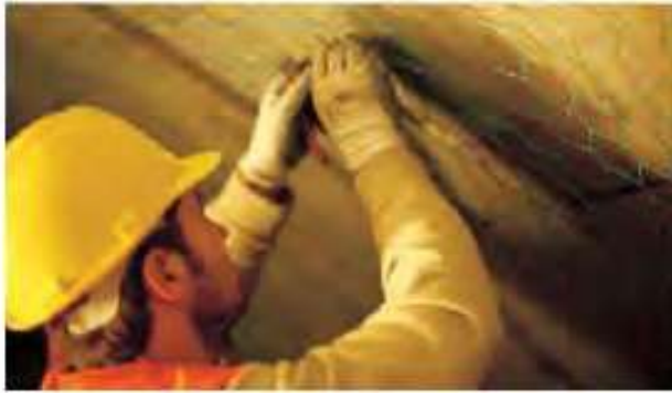
Figure 15. Mesh installation
