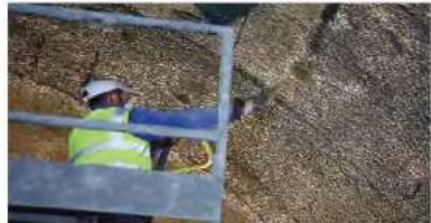
Figure 16. First coat spraying
