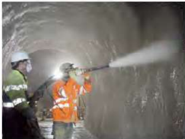
Figure 12. Manual membrane application
