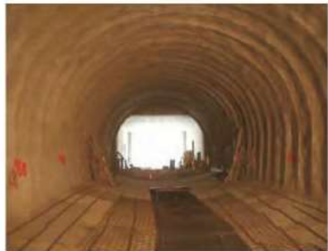
Figure 8. Tunnel section during construction
