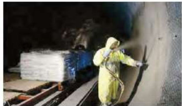
Figure 18. Regular thickness check during spraying.
