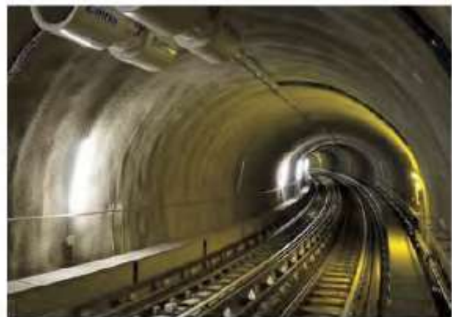
Figure 9. Final tunnel section in operation
