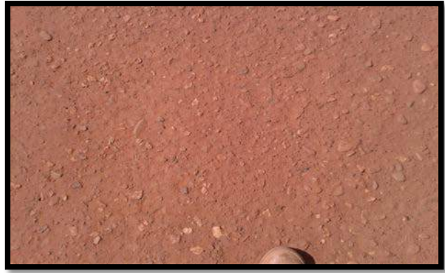
Figure IV - Gold mine haul road; Mali A. Surface after one month of traffic B. Close-up of haul road surface
