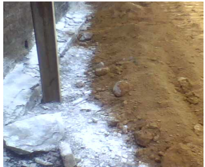
Figure 3. Fire combated portion treated with binding material with top soil near Mining workshop and Giddi power sub-station, CCL.
