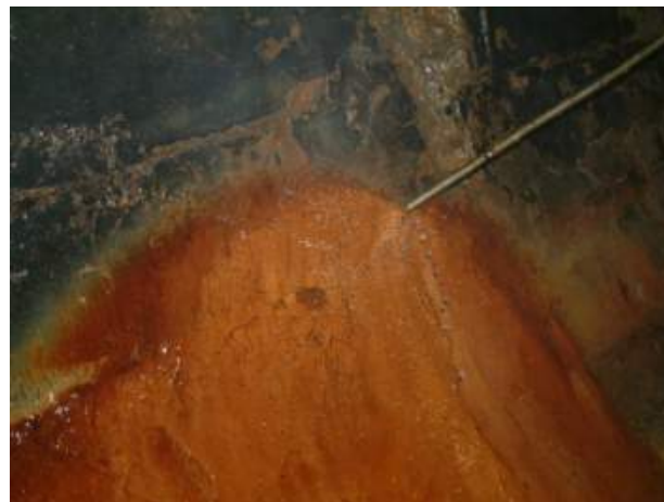
Figure 2. The appearance of concrete damages to the reinforcement in the side part of calotte
