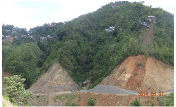
Plate 3. View of rocky portion that required blasting operation at Ch: +2150 m
