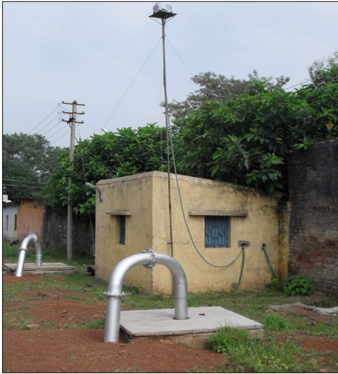
Figure 7. Pump house for two submersible pumps.
