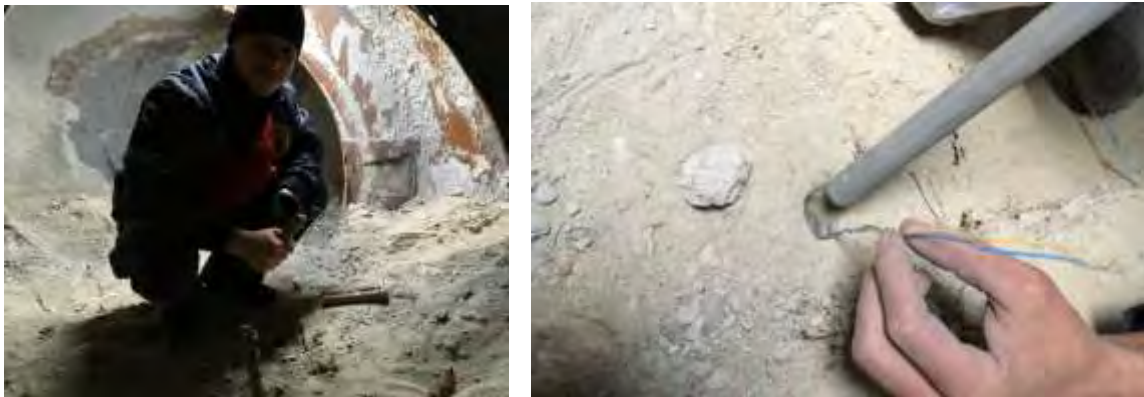
Figure 10. Loading of the charges inside the blast holes
