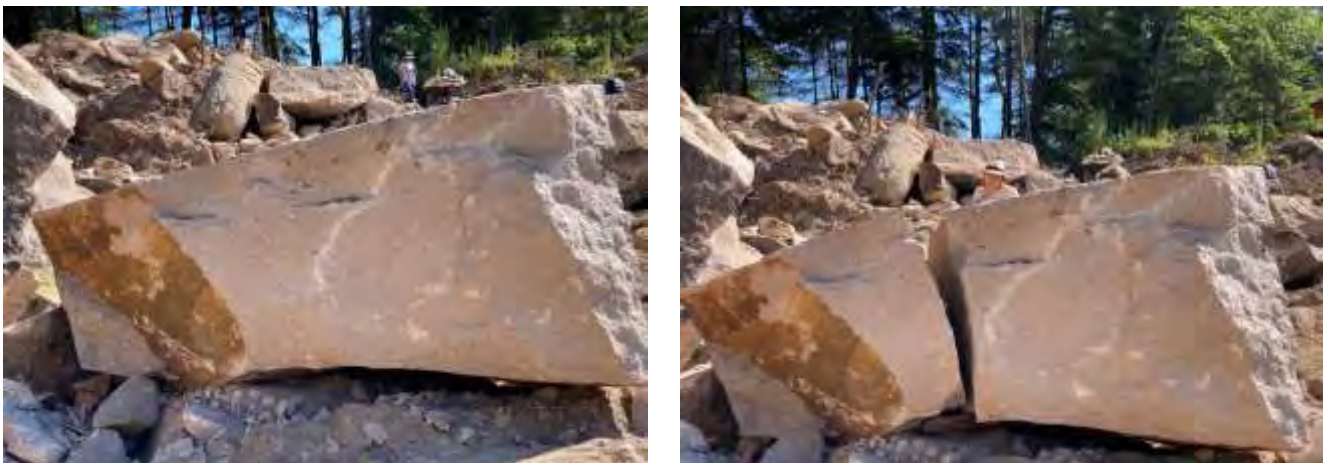
Figure 7. Splitting of a boulder with one charge of 50 g. Mixture #2 in single blasthole with length 0,60 m.
