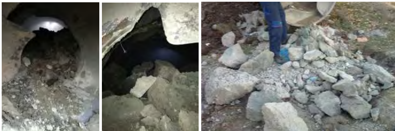
Figure 11. Fragmentation of the concrete after blasting
