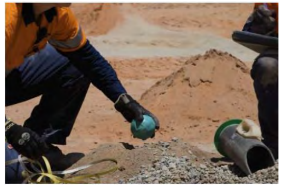
Figure 9. Placement of BMMs
