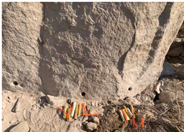
Figure 3: Ready for loading charges of propellant-based non-detonating compositions
