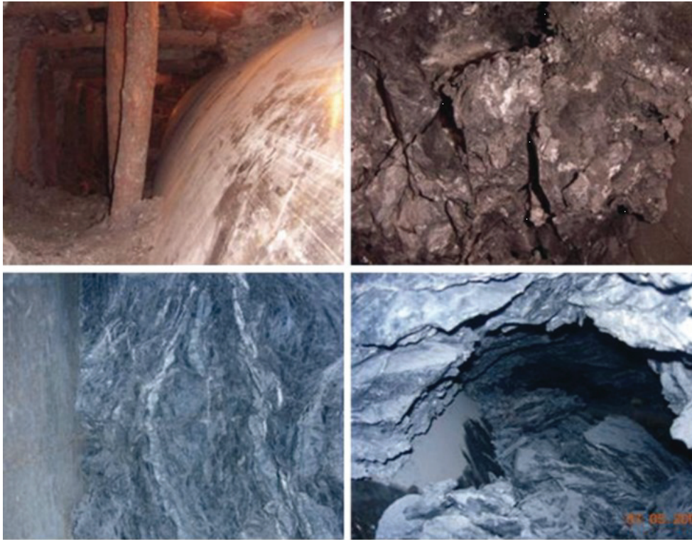
Figure 6. Rock formations in Uluabat Tunnel and trpped TBM
