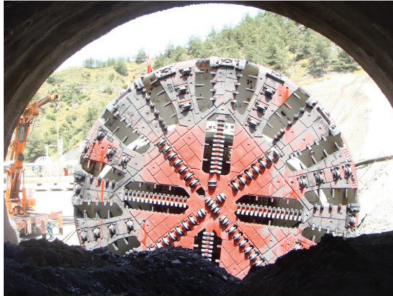
Figure 2. 13.7 m diameter single shield TBM used in the project
