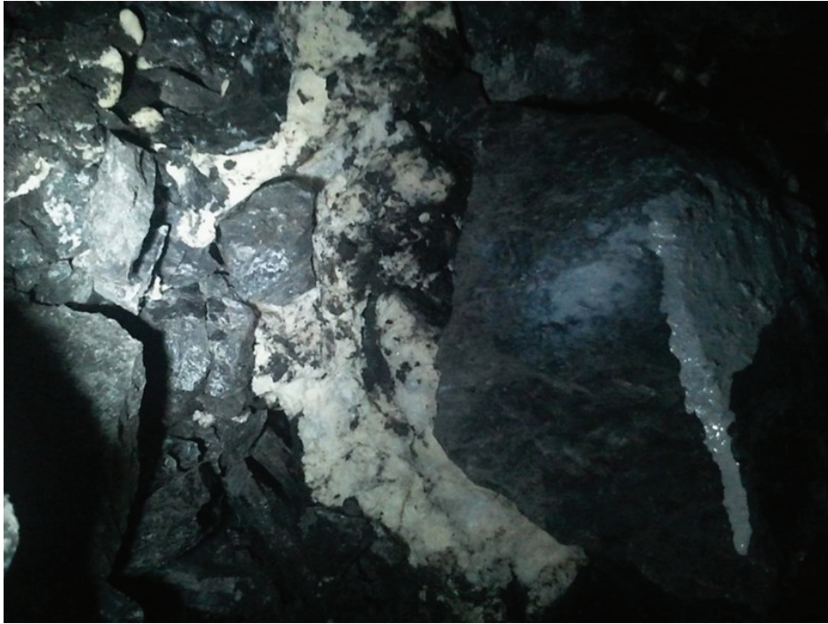
Figure 13. Polyuretane injection to stabilize the tunnel face in Kargı Tunnel
