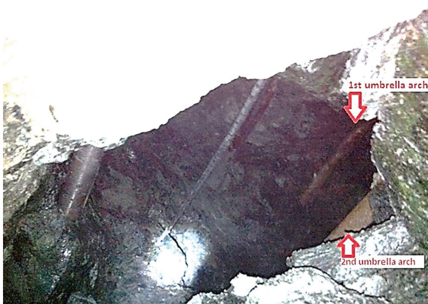
Figure 14. The application of umbrella arch in Kargı Tunnel
