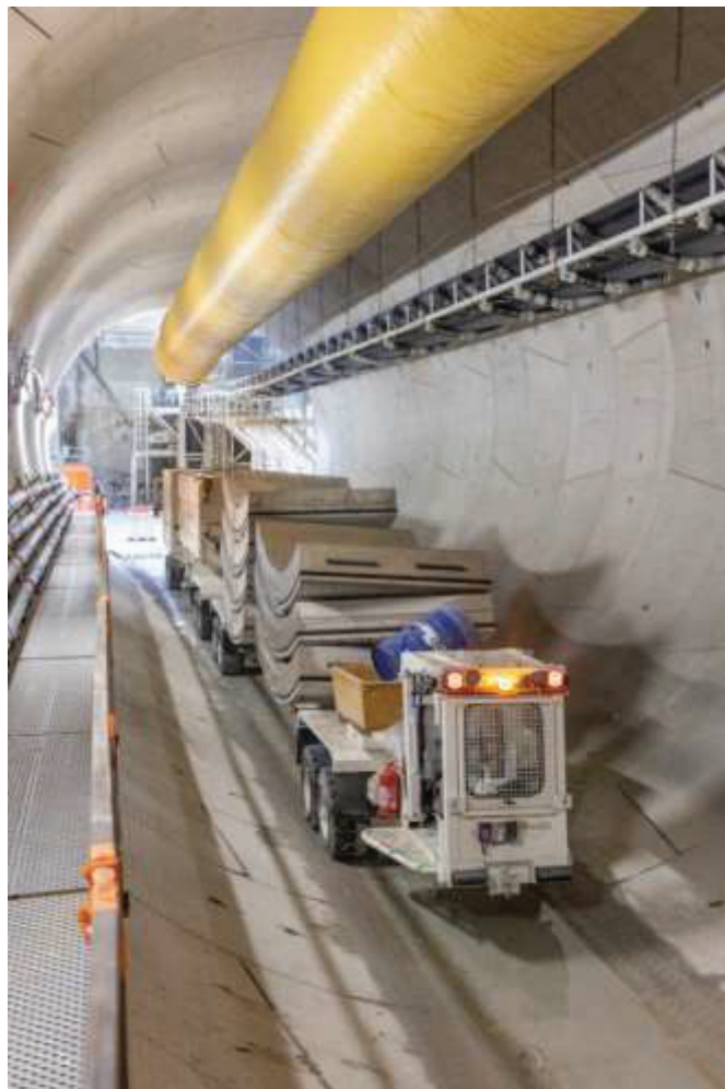
Figure 4. Project jobsite Grand Paris - Photo Credit Eiffage Génie Civil.
