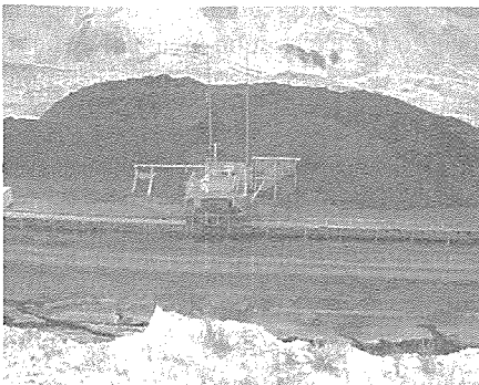
Figure 12. Reclaim feeder / breaker.
